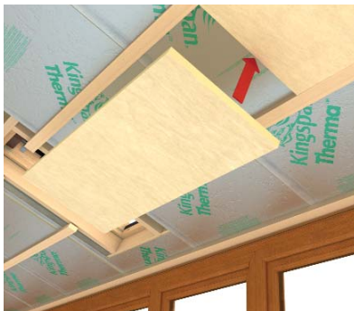
Install insulation between batten
